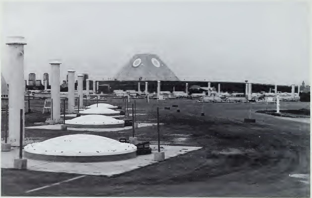
Fig. 2-37. The SAFEGUARD site became the western world's only operational ABM site. The MSR and its missile silos stand ready to protect the nation.
